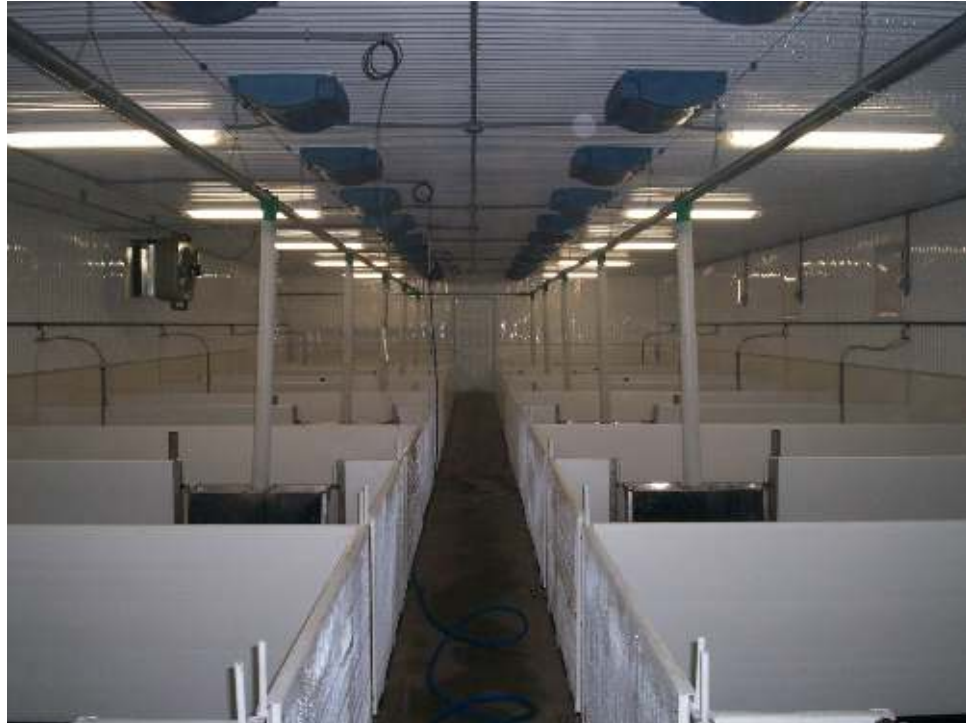
Figure 6: Example of ceiling inlet installation
