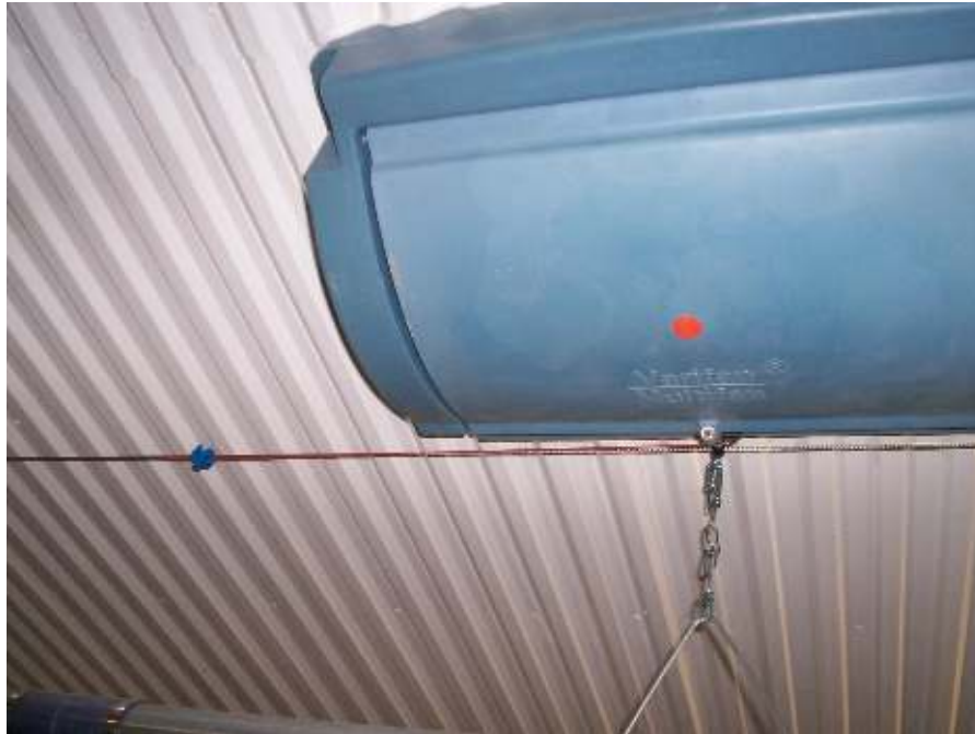
Figure 7: Connection example of the air inlet and cable
