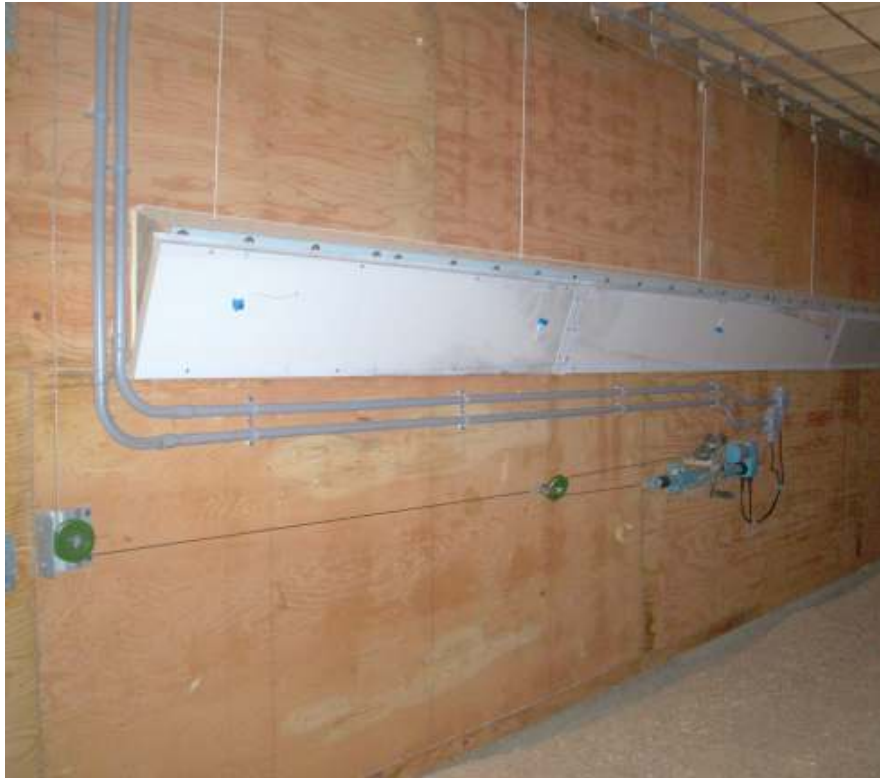
Figure 9: Another example of an air inlet installation on a wall
