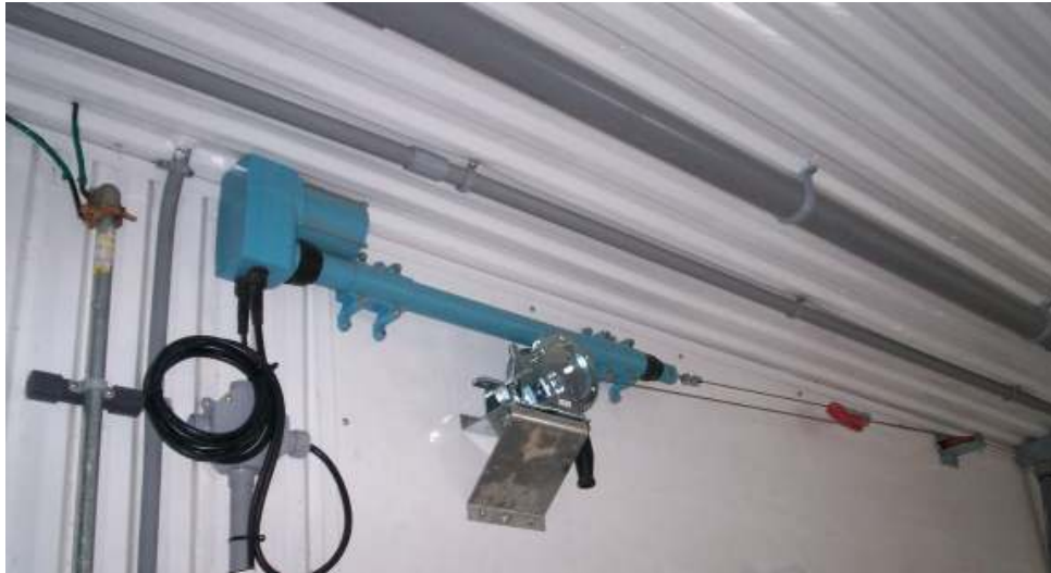
Figure 5: Example of winch, pulley and actuator installation
