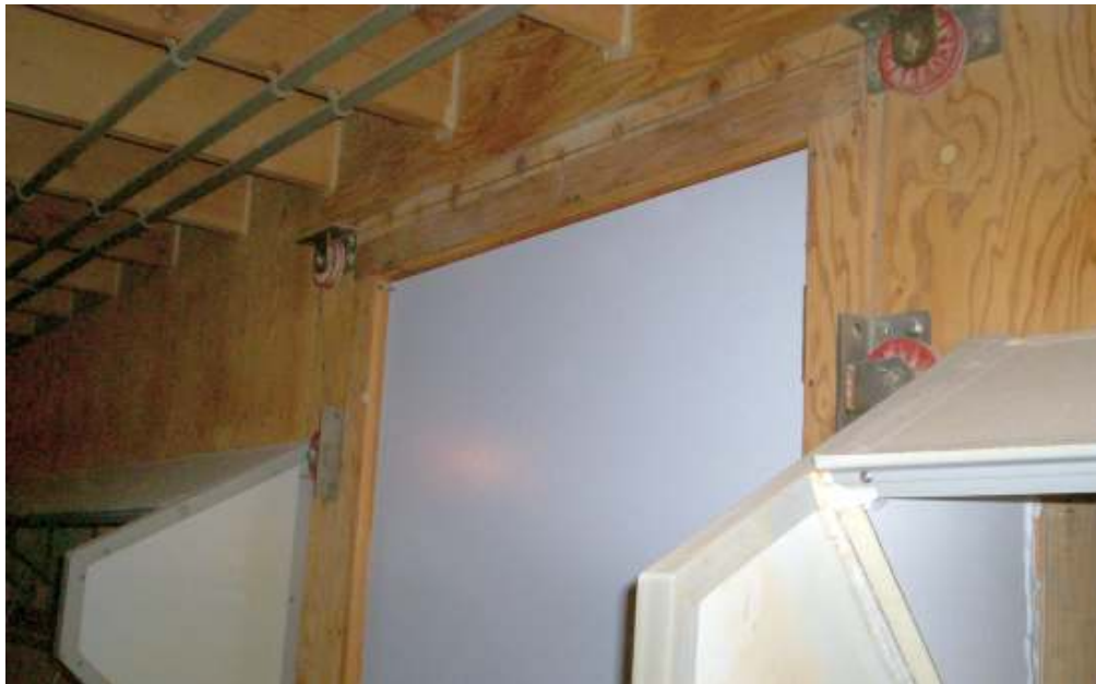
Figure 14: Example of an installation avoiding an obstruction (a door)
